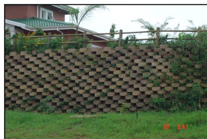
DRY STACK RETAINING WALLS
