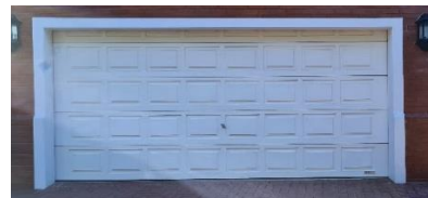
Existing Raised and Fielded
